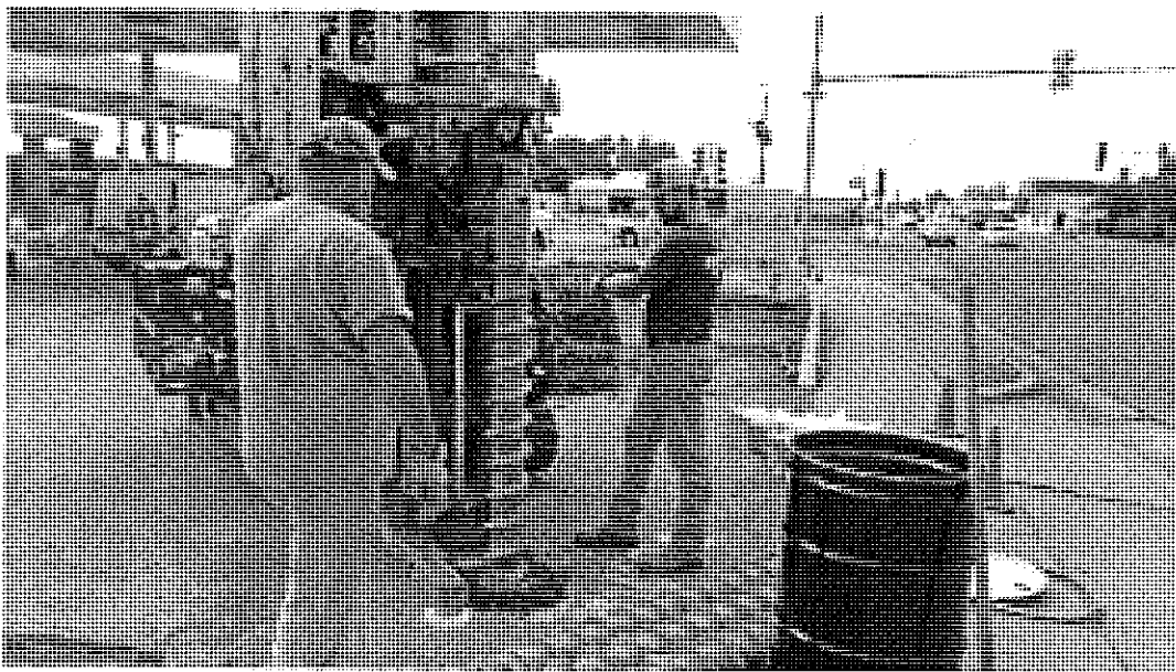
PROJECT: Johnson Oil Company-Danville PHOTOGRAPH #20 DATE: 7/20/23 VIEW: South DESCRIPTION: Drilling Monitoring Well PMW-20.
