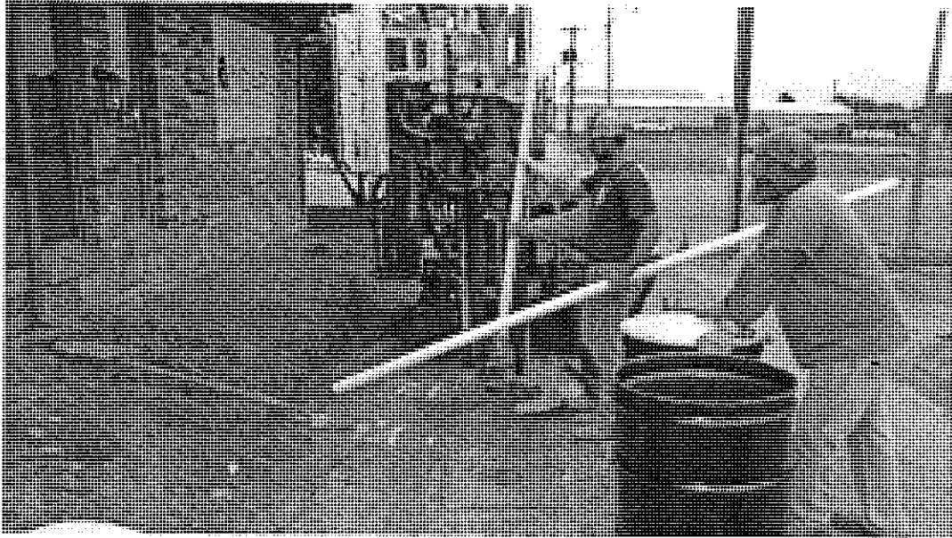
PROJECT: Johnson Oil Company-Danville PHOTOGRAPH #13 DATE: 7/20/23 VIEW: South DESCRIPTION: Installing Monitoring Well RMW-13.
